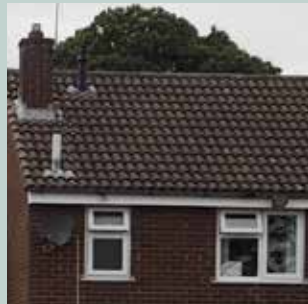
Glazed pantile roof
