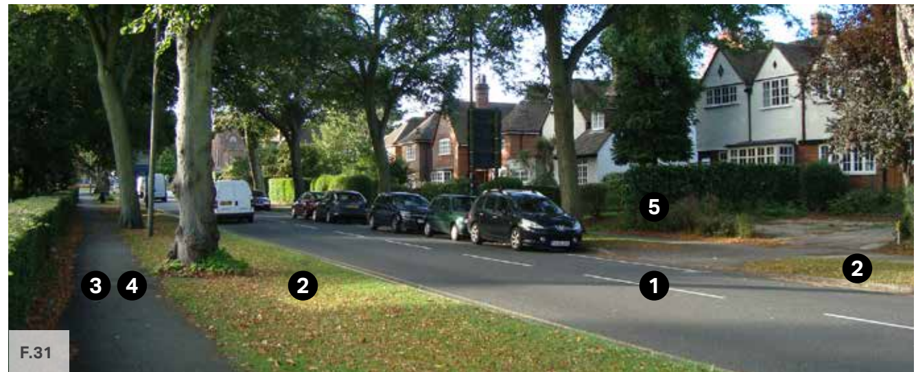
Figure 31: Primary road usually framed by wide tree verges shown on above section in a residential neighbourhood. It is recommended that cycle provisions are separated from moving traffic and that parking bays, where required, are inset into the verges to avoid impeding the movement of pedestrians and vehicles. Long Street is a primary road as the main arterial road run through south to north.
