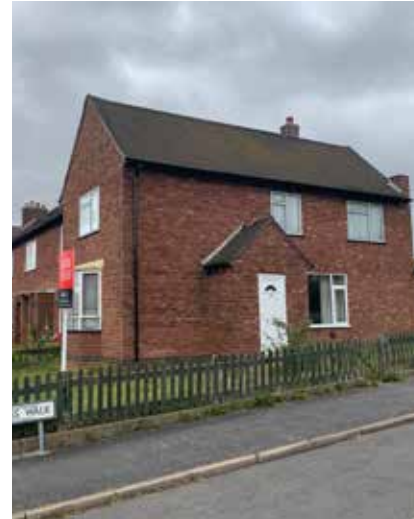
BU 09. Corner buildings
