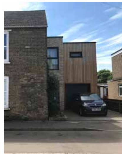
BU 12. Extension & alteration
